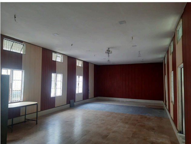
Constructing ICT classrooms
