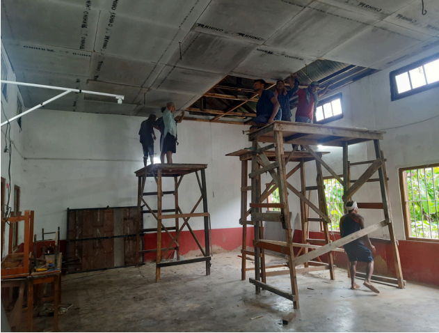
Repairing the roofs in classrooms
