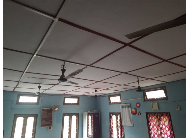
Installing the ceilings in classrooms
