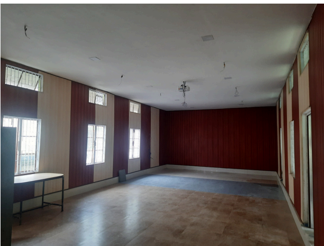
Constructing ICT classrooms
