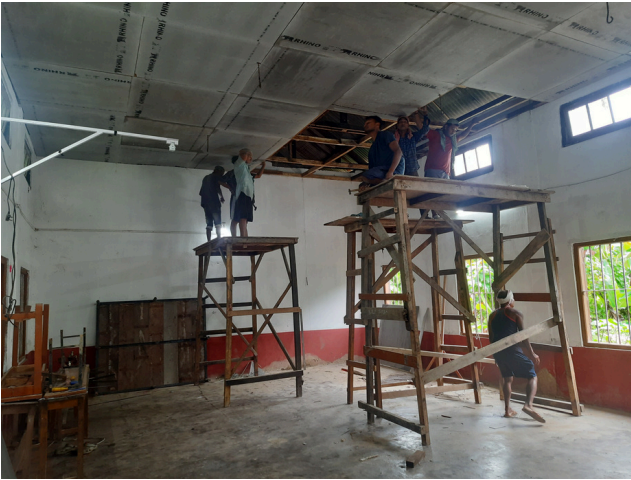
Repairing the roofs in classrooms
