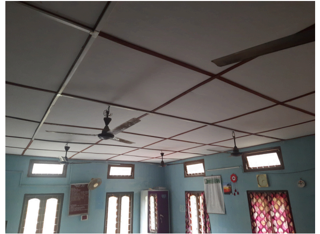
Installing the ceilings in classrooms
