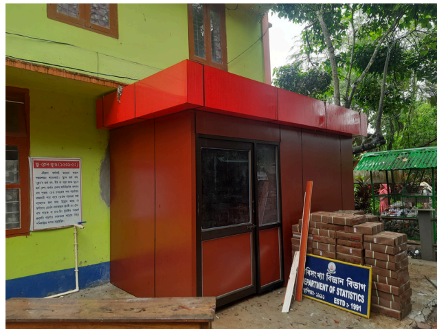
Constructing drinking water facilities
